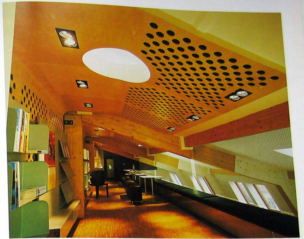
The simultaneously-installed holes in the birchwood ceiling are a structural design element. Built-in spotlights by Zumtobel Staff. ■
