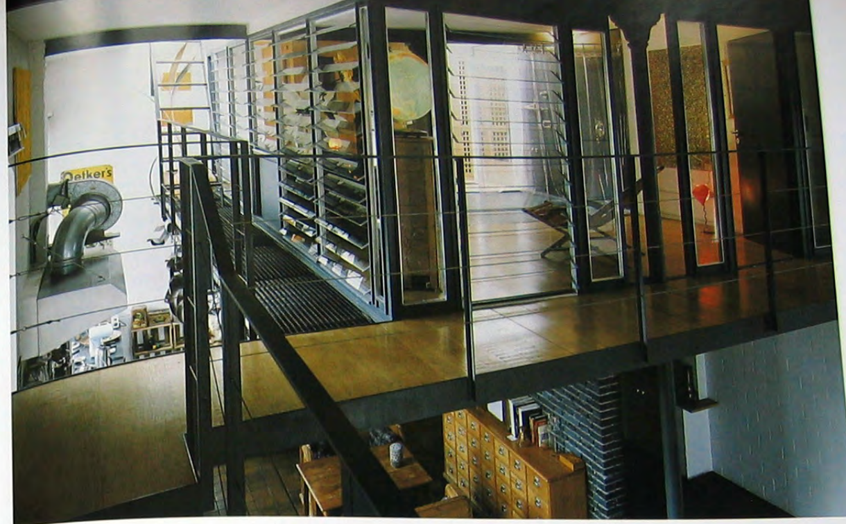
The steel girders form galleries and bridges and link the various living and working areas. In front, the sauna. ■
